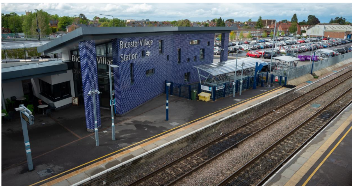
Figure 27 – Photo of Bicester Village Station which was delivered during Phase 1 of East West Rail
